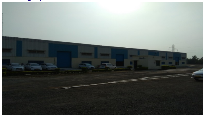
Exhibit 5: Procurement center and warehouse in the Choupal Saagar premises
