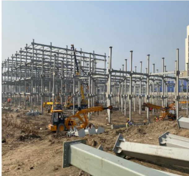
Hospital structure put in place in 6 weeks
